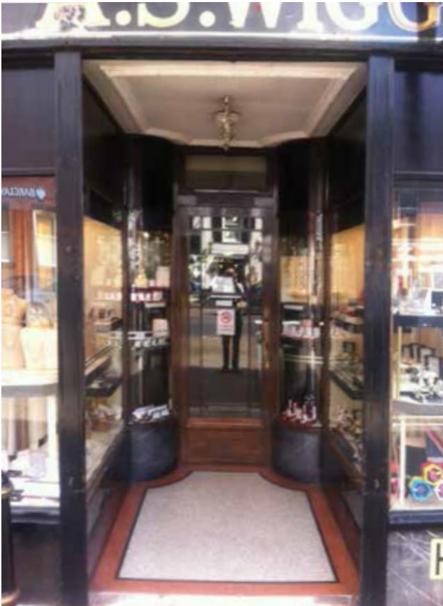
Well designed entrance: recessed, level access and outward opening
